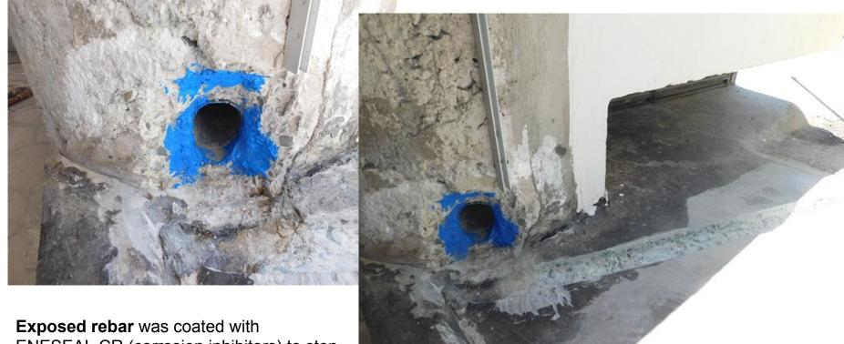
**Exposed rebar** was coated with ENESEAL CR (corrosion inhibitors) to stop further corrosion of metal.
