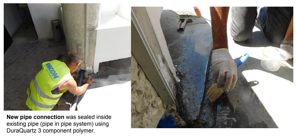
**Area** to accept new pipe is primed with 2 component polymer for excellent adhesion.
